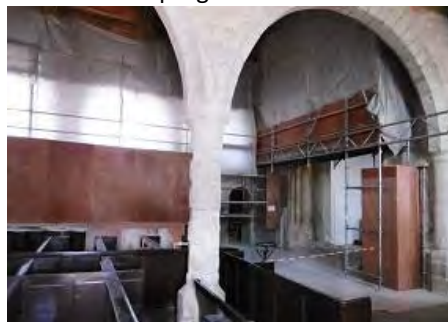
The work in progress at the church...
